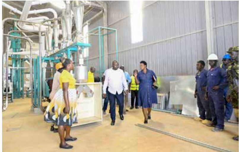
State House Comptroller inspects the installation of Maize Value Addition plant at Bunyoro Zonal Presidential Industrial Hub in Masindi on 20 th October 2025.
