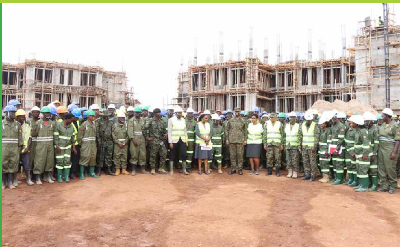
CDF Gen Muhoozi Kainerugaba with Senior Defence and UPDF officials during the site inspection of the ongoing construction works for the Joint MoDVA/UPDF Hq in Mbuya
