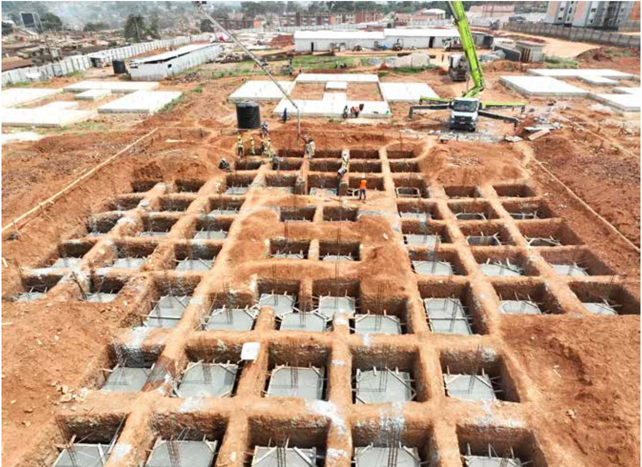
New Commissioned Construction Site of additional Housing Units at Naguru Police Barracks in Kampala.
