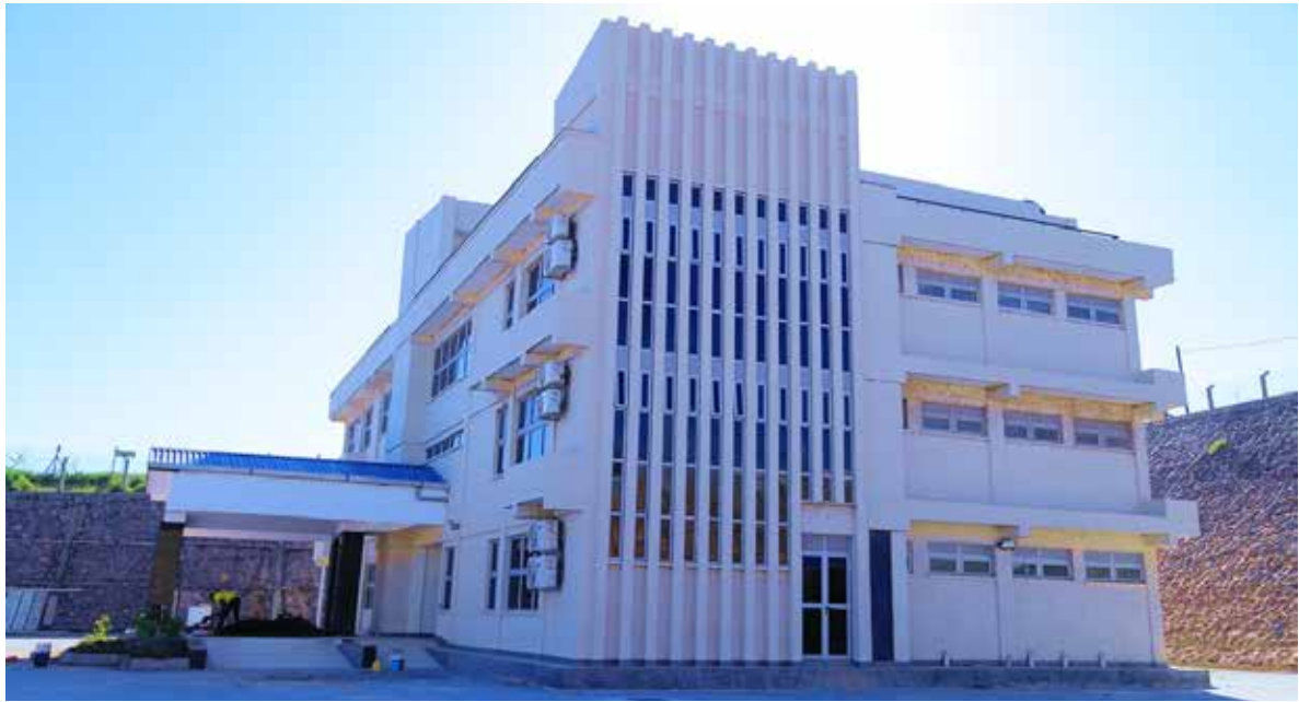
The Trade House at Entebbe International Airport Free Zone
