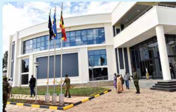
National Command and Control Centers at Police Head Headquarters Naguru.
