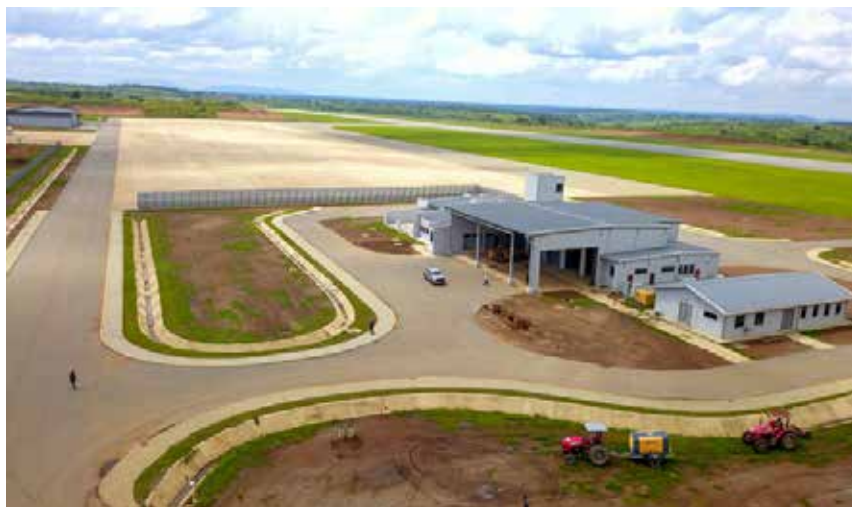
Kabalega international Airport in Kabaale village, Kabaale sub county in Hoima. The handover of the airport has been pushed to September 2025.
