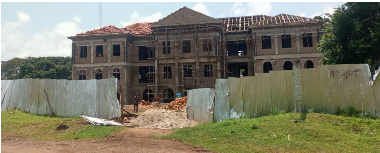
The construction site for Tororo High Court Building.
