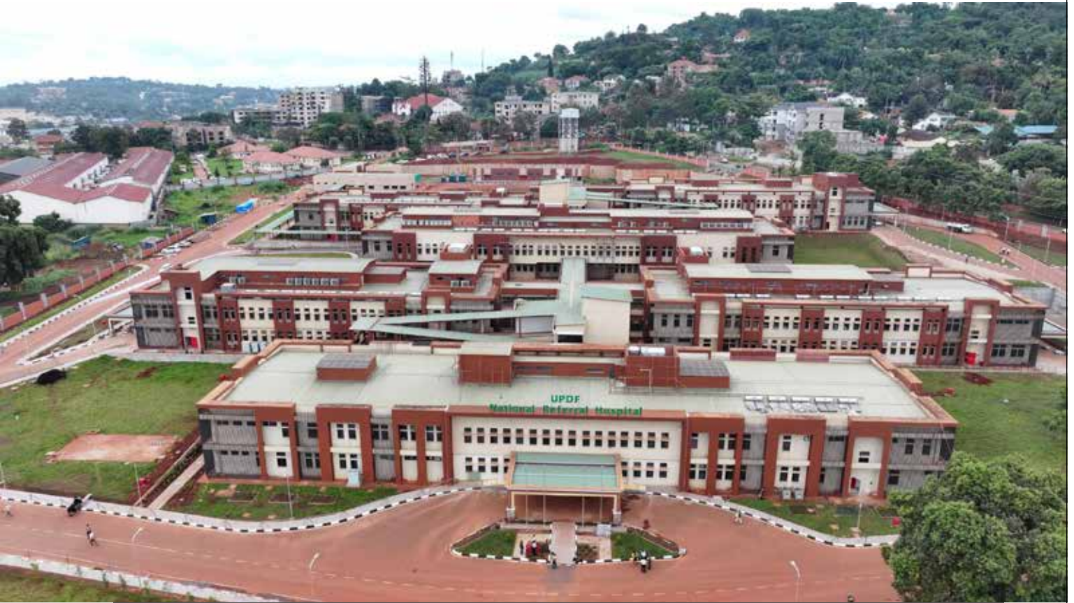
An aerial view of the UPDF National Referral Hospital - Mbuya (Nakawa Division)
