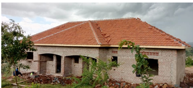
Bukwo Staff Residence
